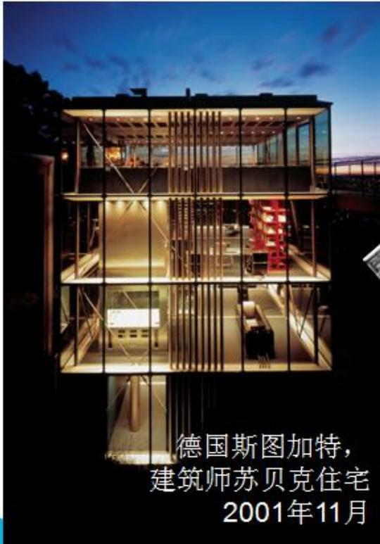
in Murr, near Stuttgart. The home's "intelligent façade" is made of a new high-tech glass containing a metal-coated plastic film and two layers of argon gas. The outer sides of the glass are invisibly coated with metal microns.
